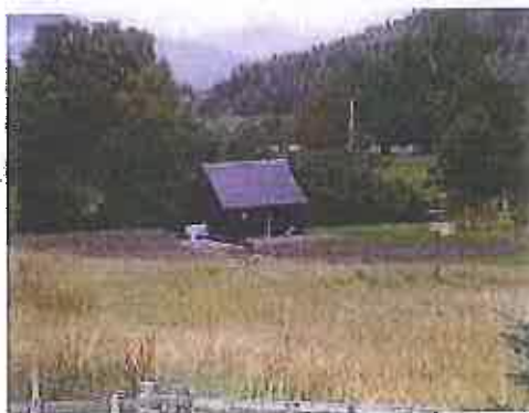
Figure 4 – a powerhouse for a 99kw turbine
